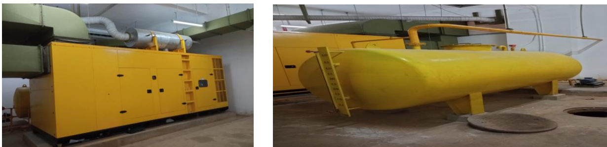
Biodiesel Generator and Power Integration Unit (Esa Unggul University – Cikupa - Tangerang) Esa Unggul University – Cikupa- Tangerang already has a renewable energy source, namely BIO DIESEL with a capacity of 640Kwh that reaches the entire building area as well as the main street lights.
