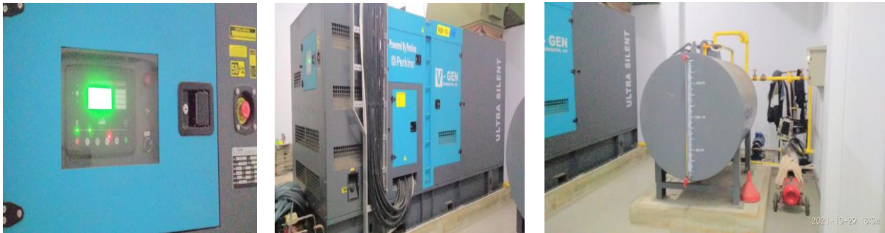
Biodiesel Generator and Power Integration Unit (Esa Unggul University - Bekasi) Esa Unggul University – Bekasi already has a renewable energy source, namely BIO DIESEL with a capacity of 520Kwh that reaches the entire building area as well as the main street lights.
