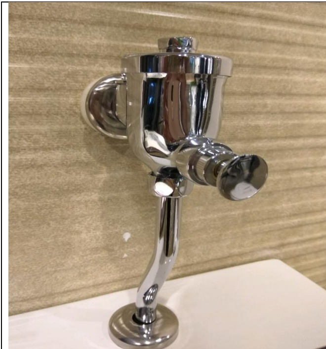
Example of Water Efficient Appliances Usage Flush Valve Urinoir (Esa Unggul,Indonesia)
