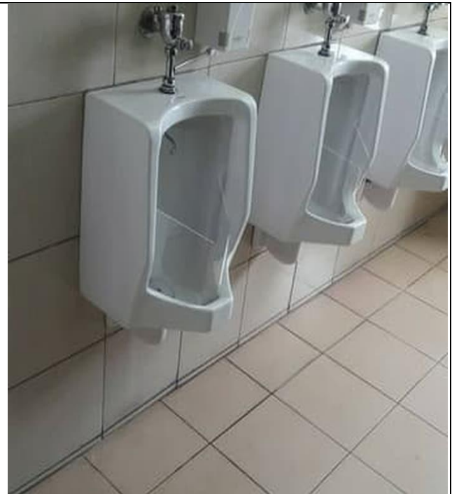
Example of Water Efficient Appliances Usage Flush Valve Urinoir (Esa Unggul,Indonesia)
