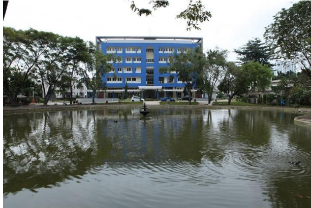
Water Conservation – Rain Water Collection (University of Esa Unggul, Indonesia)
